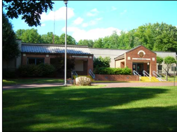
Richland Township Municipal Building
