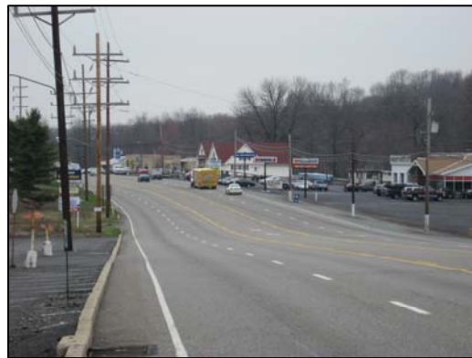
Commercial Corridor along Route 309
