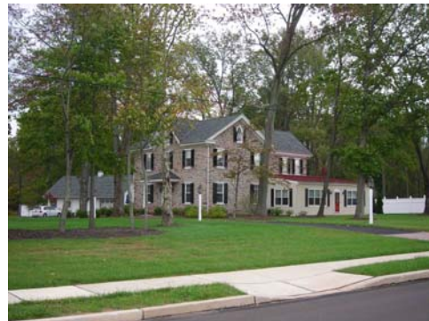
Refurbished House Adjacent to a New Residential Development
